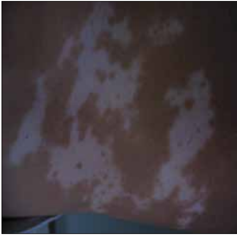
Figure 4: Control site (before treatment)
